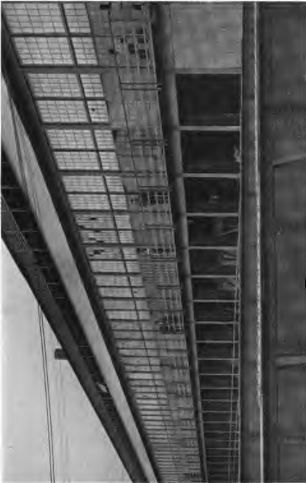
Fig. 1. Footwalk on Outside of Open-Hearth Building, giving access to Crane Runway within. (American Steel and Wire Company.)*
